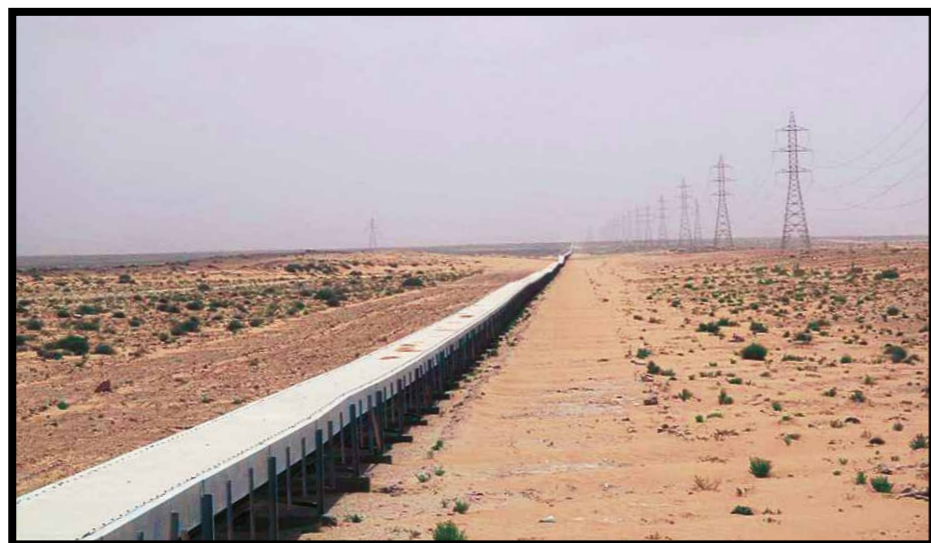
The Moroccan conveyor belt for phosphates from the occupied Western Sahara is more than 100 km long and thereby the world's longest.
