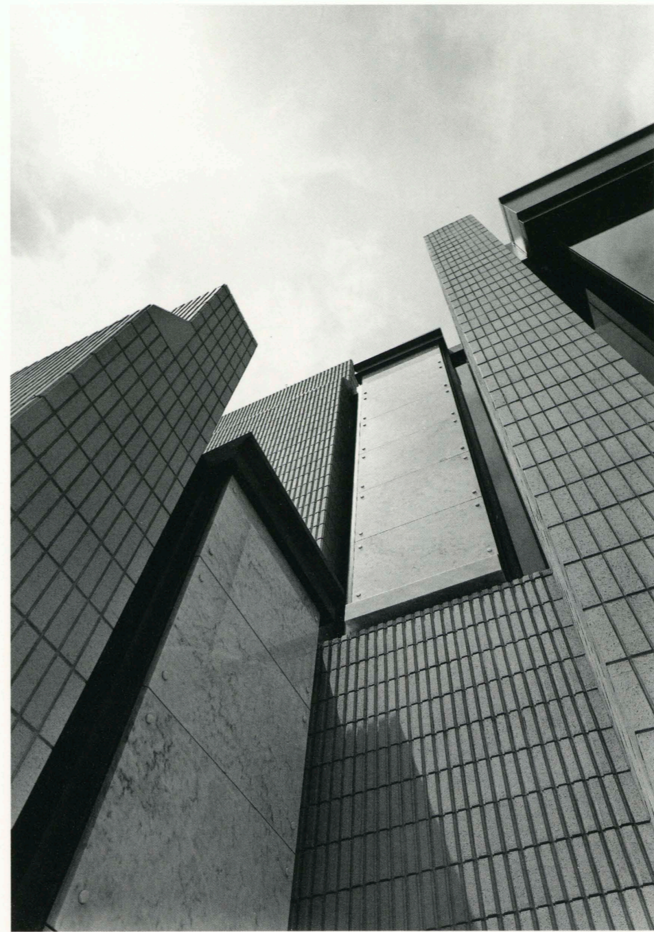
外観見上げ Upward view of the exterior.
