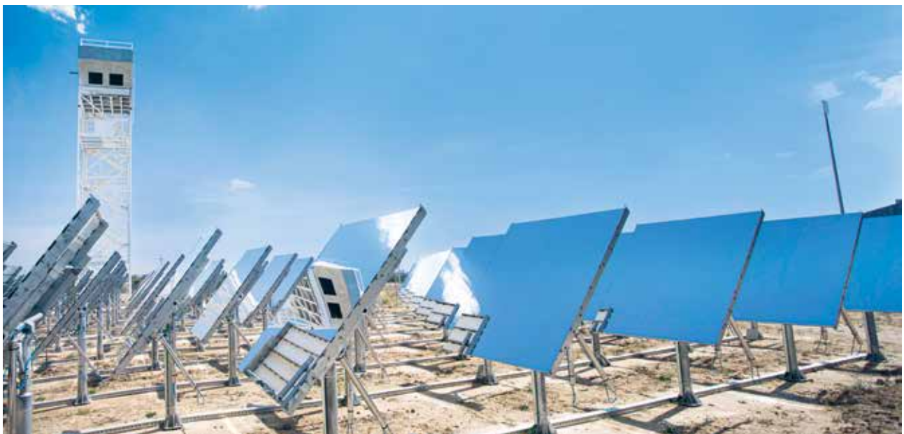
Sun-to-liquid (StL) process — A sun-to-liquid plant produces kerosene from sunlight, water and CO 2 . The process is already in use: in Madrid, the IMDEA Energy Institute built a unique solar facility and tested it extensively over four years. MTU was involved in the project as a member of Bauhaus Luftfahrt, the German aviation industry's think tank, which was responsible for the entire technology and systems analysis. The challenge now is to scale up the production process.
