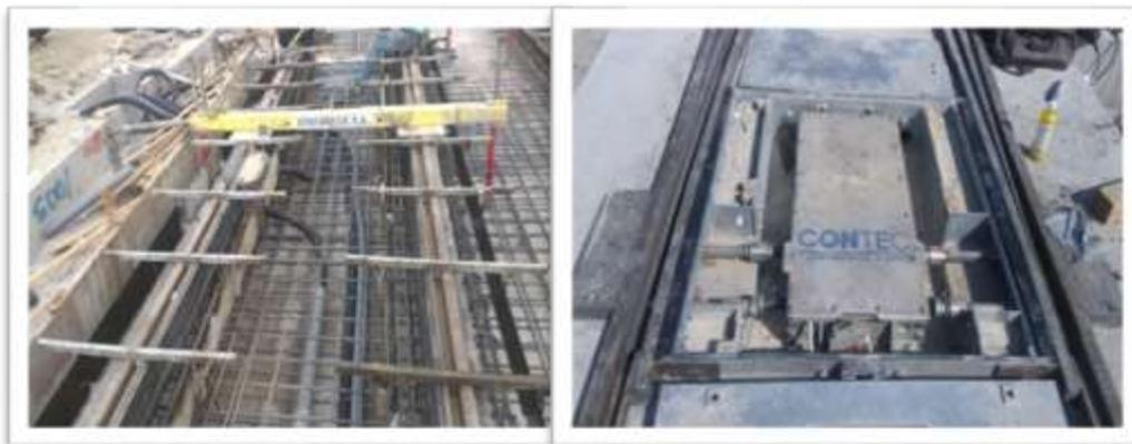
計軸器、轉轍器安裝施工
