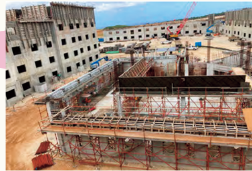
Progress of the Building Development Project for Non-commissioned Officers in Finegayan
