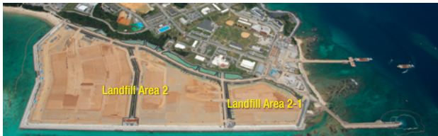
Progress of landfill work
