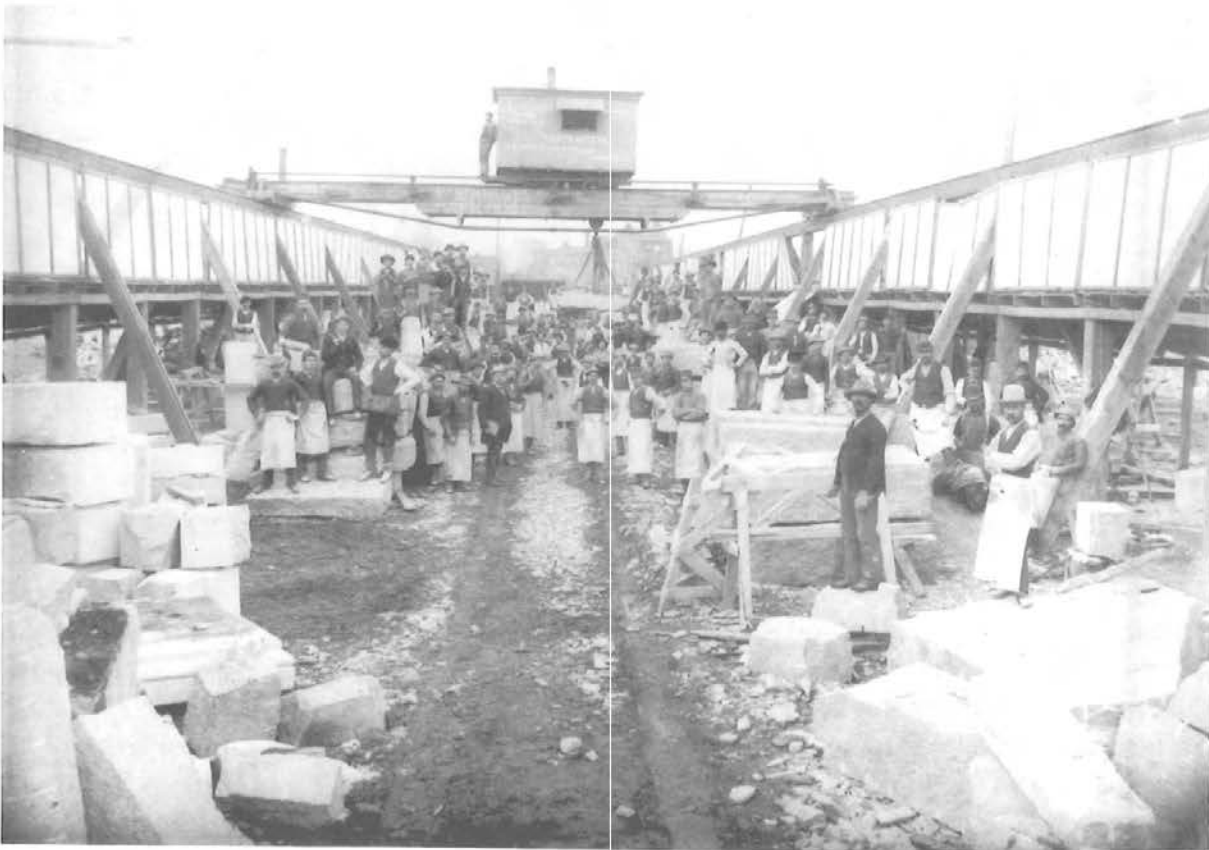
Figure 2. Stone cutters in Denver finish blocks of Aberdeen granite for the Colorado state capitol building. Colorado Historical Society.
