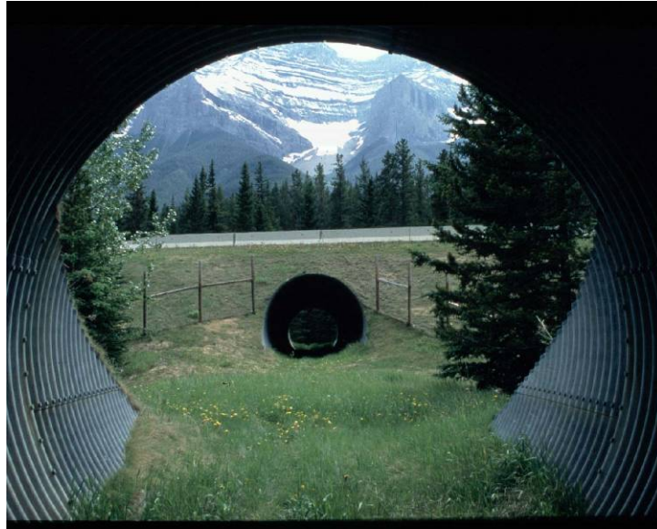
Figure 25. A large wildlife crossing culvert. Photo by Tony Clevenger, WTI.
