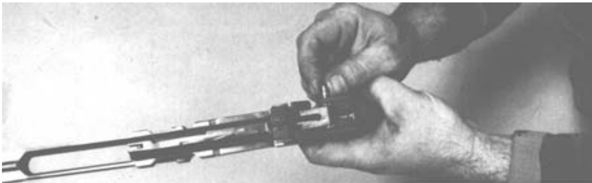
Step 1. Removing the Spring Loaded Pin.
