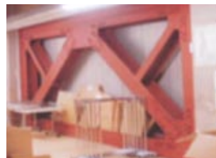
Reinforcement by steel frame braces
