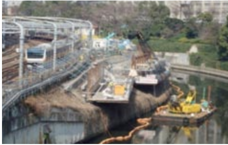
Seismic reinforcement of embankment
