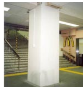
Reinforcement of columns by steel plate wrapping
