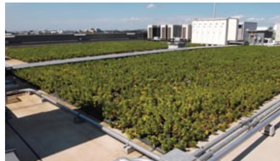
Rooftop greening at the Chiba branch building
