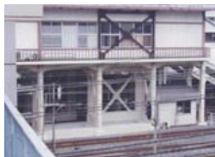
Reinforcement by steel frame braces
