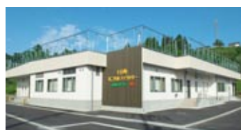
Tokamachi Sukoyaka Factory
