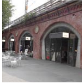
Brick arched elevated bridge
