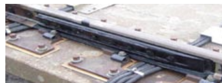
After improving glued insulated joints
