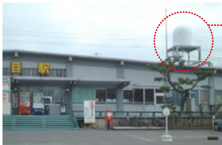
Doppler radar installed on the roof of Amarume Station on the Uetsu Main Line
