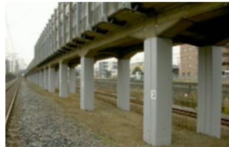
Seismic reinforcement of elevated bridge columns by steel plate wrapping
