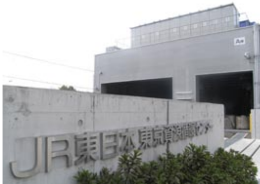
JR East Tokyo Materials Recycling Center
