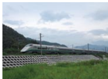
Embankment slope protection (spray frame work)
