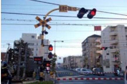
A crossing warning device located in a higher position for better visibility
