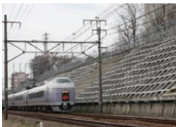
Cutting slope protection (spray frame work)
