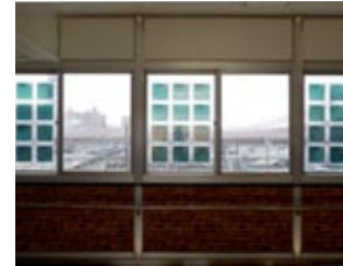
Organic thin-film solar cells on overpass for transferring passengers (Fukushima Station)
