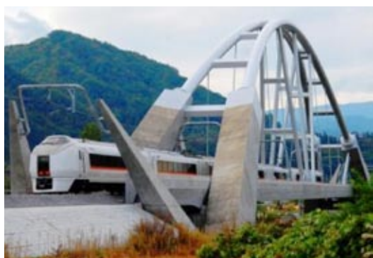
Agatsumagawa Bridge No. 3
