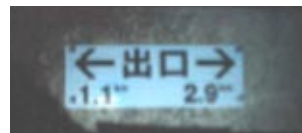
Sign to indicate distance to a tunnel exit
