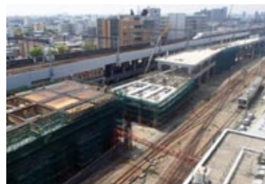
Railway overpass construction project near Niigata Station on the Shin-etsu Line
