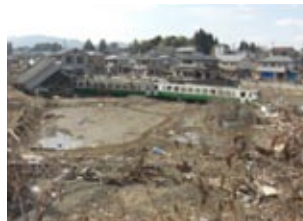
Kesennuma Line, between Saichi and Matsuiwa, 2942D
