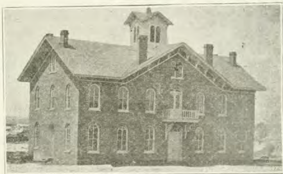
COLORADO SEMINARY, 1864 First building of Denver University
