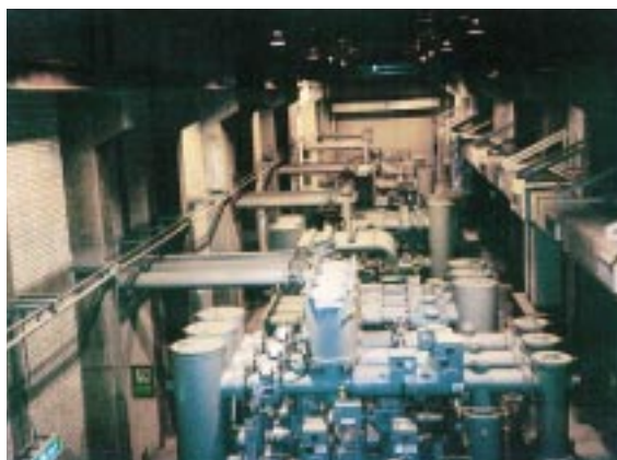
245 kV GIS 245 kV gas-insulated switchgear for ANSDK
