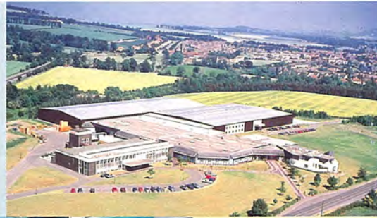
◀ Livingston Factory, Mitsubishi Electric UK Ltd.
