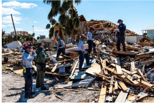
FEMA Urban Search and Rescue Task Force searches through destroyed homes looking for survivors in Mexico Beach Fl, after Hurricane Michael made landfall.
