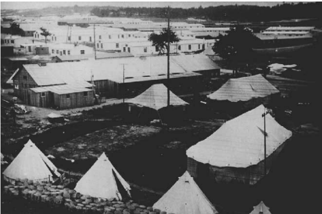
Fig. 1. The huge military camp and hospital base at Etaples.
