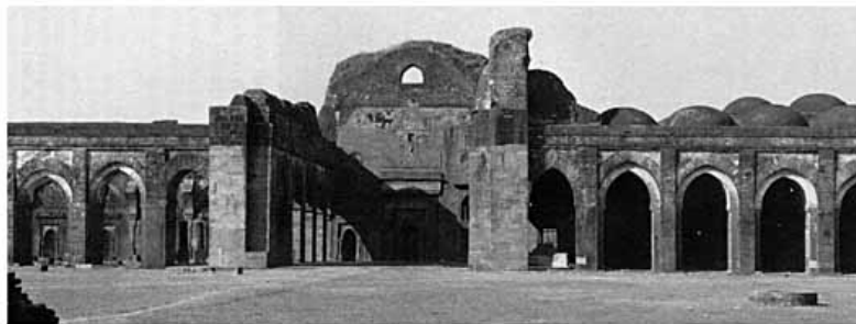
Fig. 6. Interior of Adina Mosque, Pandua (1375). Interior facing western wall, showing collapsed barrel vault. Photo by Catherine Asher. [Full Size]
