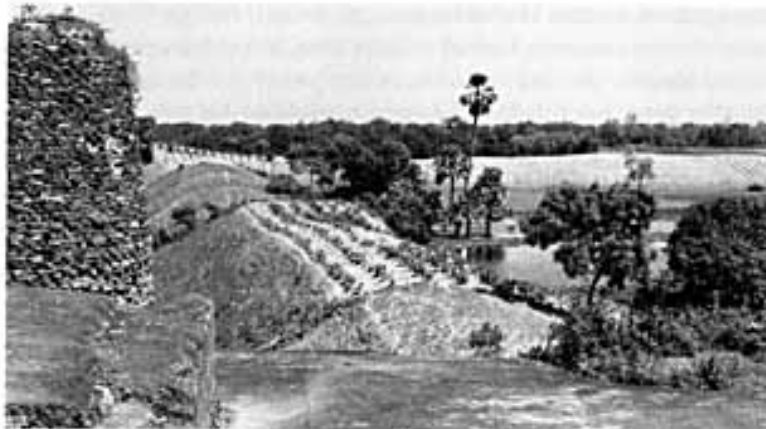
Fig. 15. Ruined ramparts of the citadel of Gaur, looking east from the top of the Dakhil Darwaza.
