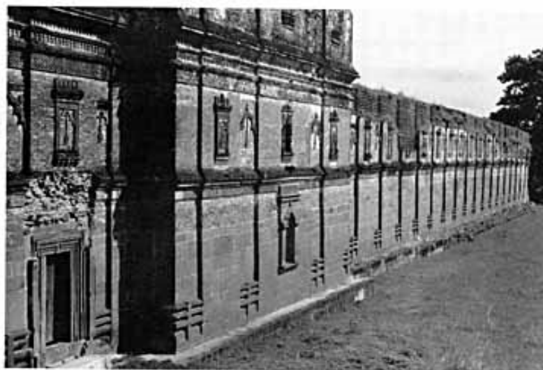
Fig. 7. Exterior of Adina Mosque, Pandua (1375). Exterior of western wall, showing facade of barrel vault. [Full Size]
