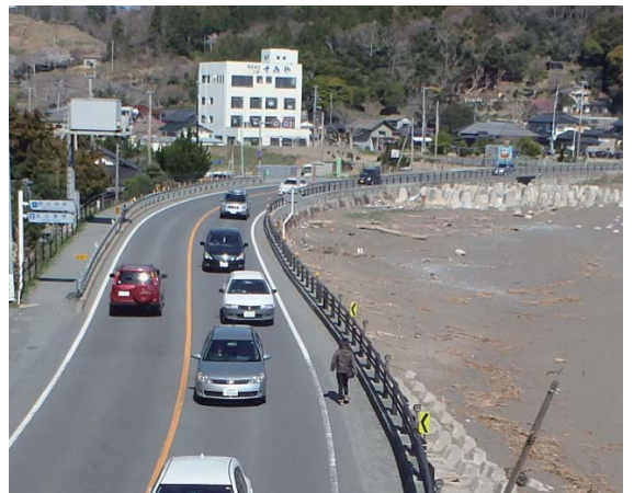
▲海側の歩道が未整備
