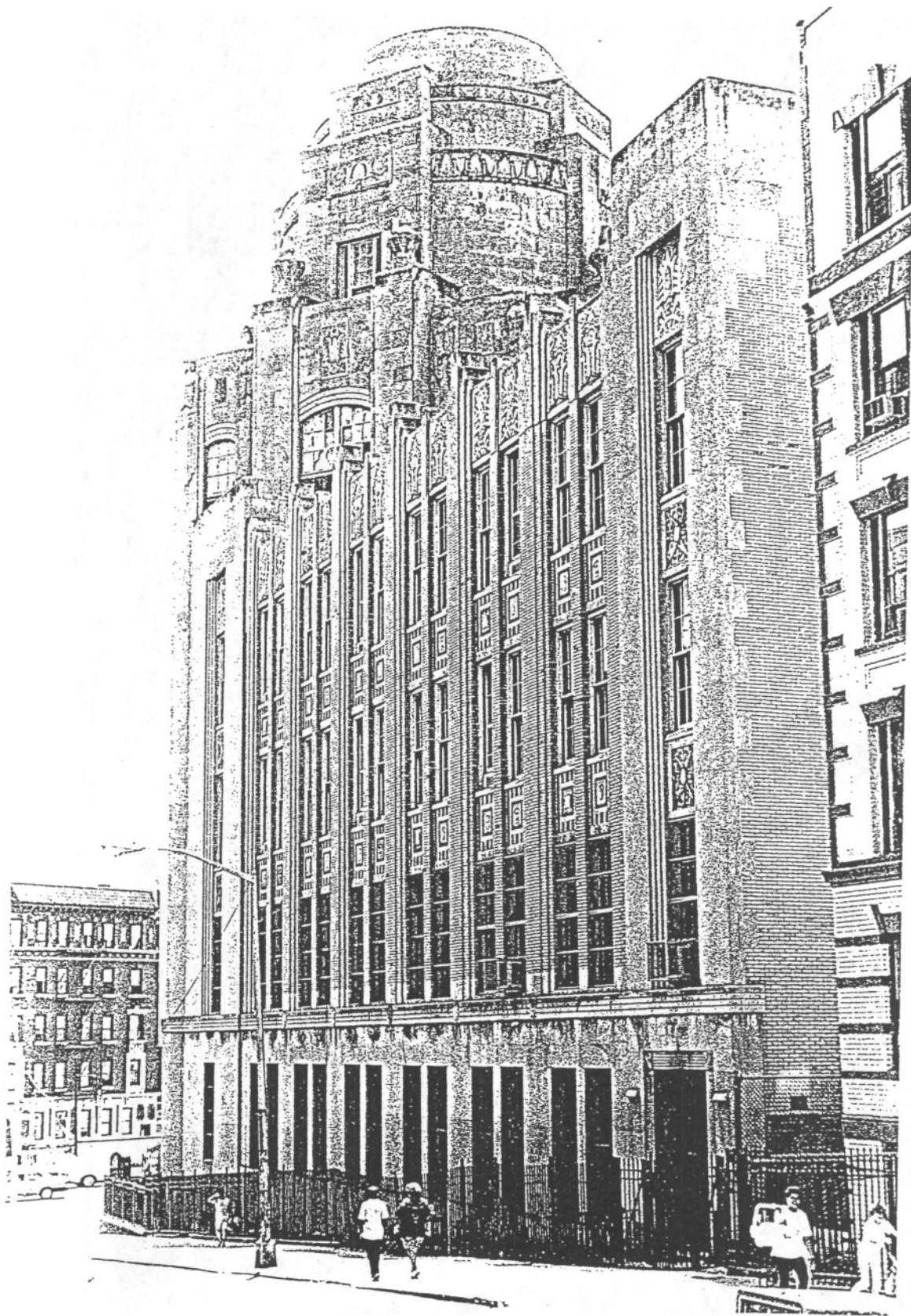
Herman Ridder Junior High School, 1619 Boston Road, the Bronx. 1929-31. Board of Education, Walter C. Martin, Superintendent of School Buildings. East 173rd Street facade. Photo credit: Carl Forster
