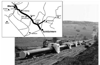
Figure 15: Pipe laying of the Ruhrgas Schlüchtern-Werne-Project Base Material - Tensile Test
