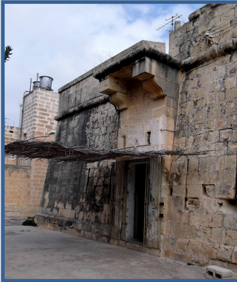
The west wall with the entrance
