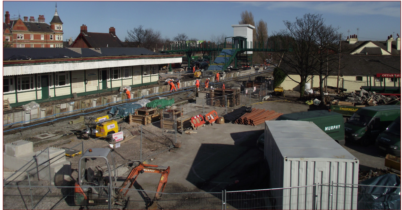
▲ Building work continues at Prestatyn as the new footbridge begins to take shape. The renovation of the station has taken well over a year and may not be completed for a further six months. The old footbridge did not accommodate easy access for those with prams or disabilities, whereas the new structure, when completed, will have long sloping ramps and a lift. Tom Peacock
