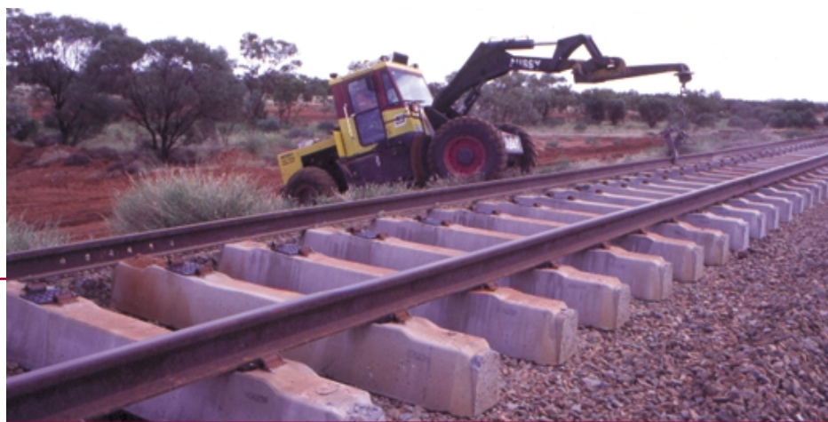
QR continues improving rail operations through upgraded infrastructure investment.
