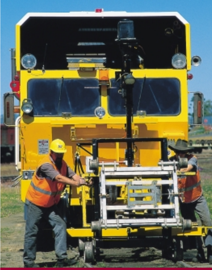
On-going track maintenance is a vital component of our train operations.
