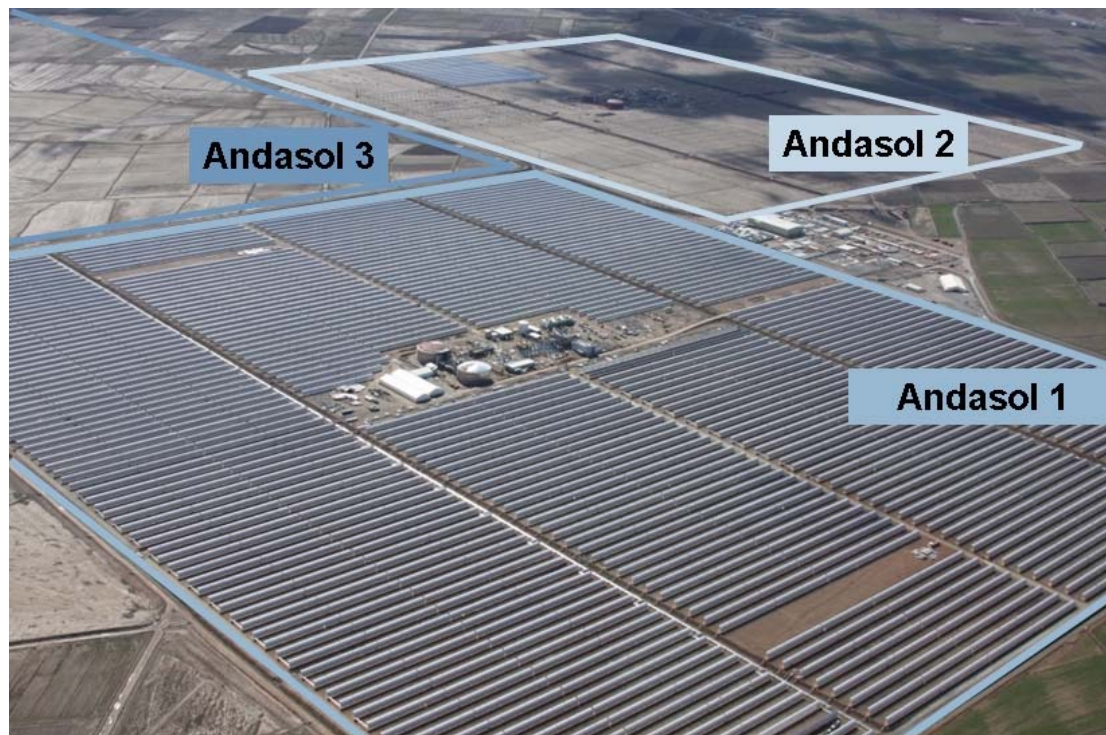
Construction site of Andasol 1 – 3 in April 2008
