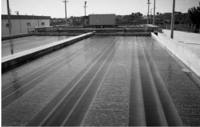
Figure - 5: Clarifiers ( Ülger, 2004 )
