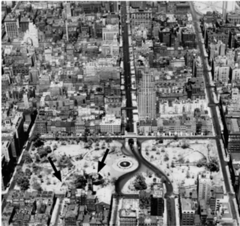
17 Aerial view 1934, looking north while the park was under construction. The Sullivan Street extension has been closed (left arrow) and the comfort station (right arrow) is either constructed or under construction. (Courtesy of Parks)
