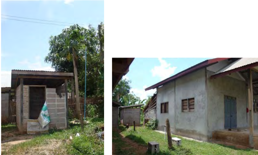
Figure 14 – Fast-track phase of UN-HABITAT project Pour-flushed toilet constructed through revolving funds and house improvements
