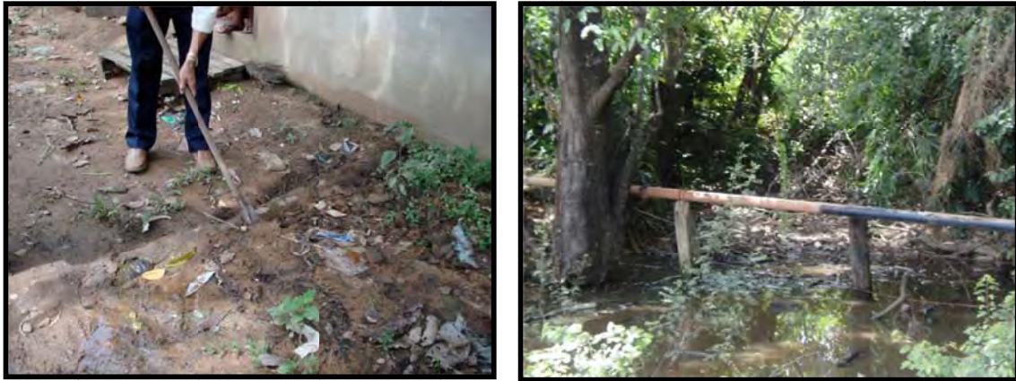
Figure 36 - Old existing distribution network
