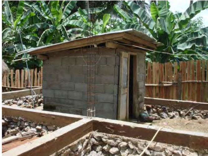
Figure 6 - Non-improved latrine in the target area
