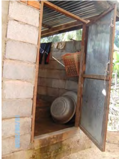
Figure 48 - Improved pour-flushed toilet in commercial sites, adapted for floods
