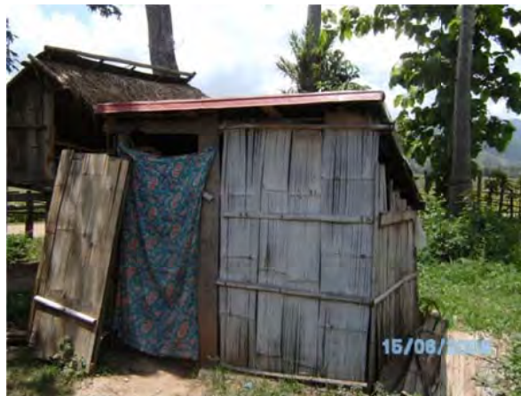
Figure 12 - Non-improved latrine in use in the target areas
