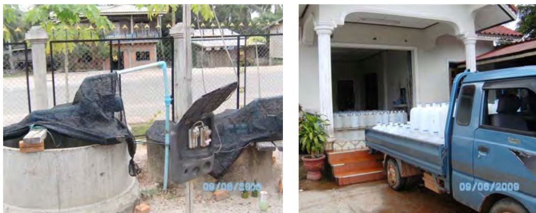
Figure 17 - Private water vendor: groundwater source and bottling system
