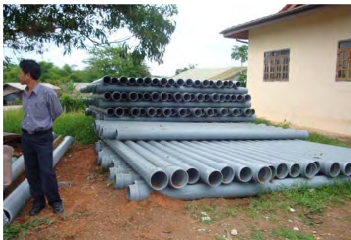
Figure 29 - New uPVC pipes for to upgrade the water supply system
