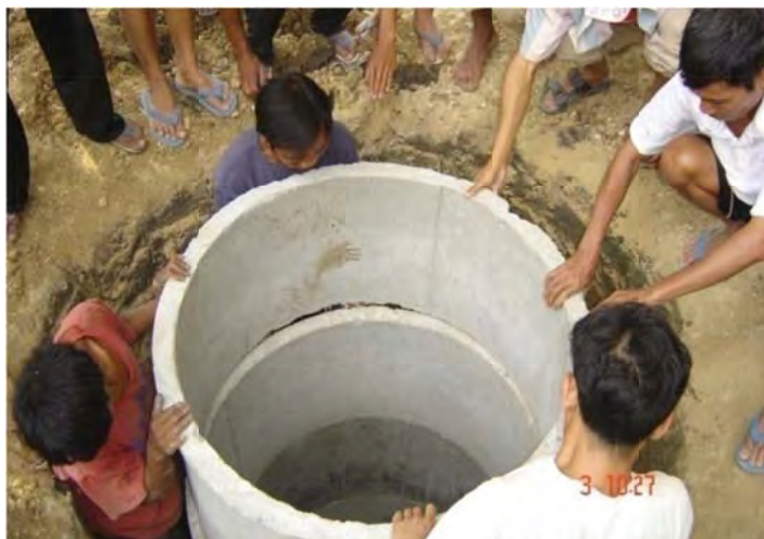
Figure 8 - Construction of lining for pour-flushed toilet
