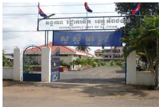
Figure 5 - KCWSU office and reservoir
