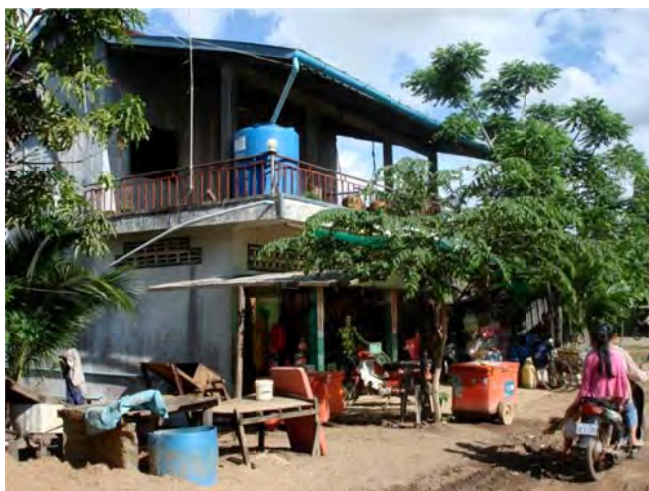
Figure 11 - Rainwater system at household level
