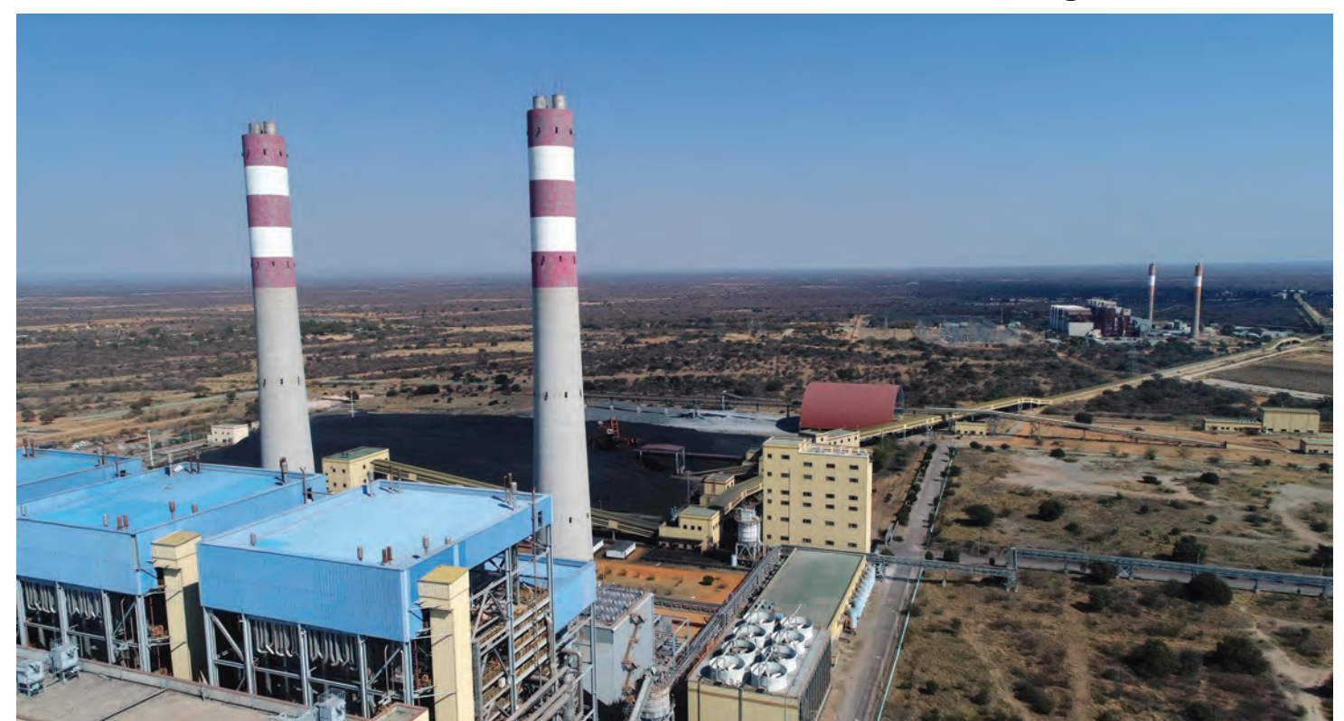
Morupule B power plant
