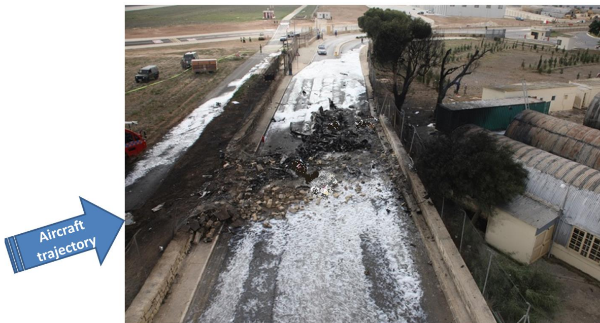
Figure 2: Damage to the perimeter wall, road and surrounding buildings
