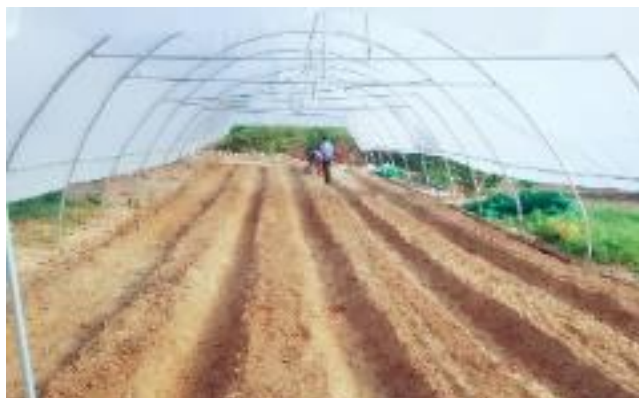
Installation of dome-shaped greenhouse underway at Nimco farm in Arabsio, [REDACTED]
