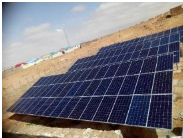
Panel set up to run two large holding freezers (40 MT) at Yustan Fisheries in Garowe. Photo credit: [REDACTED]
