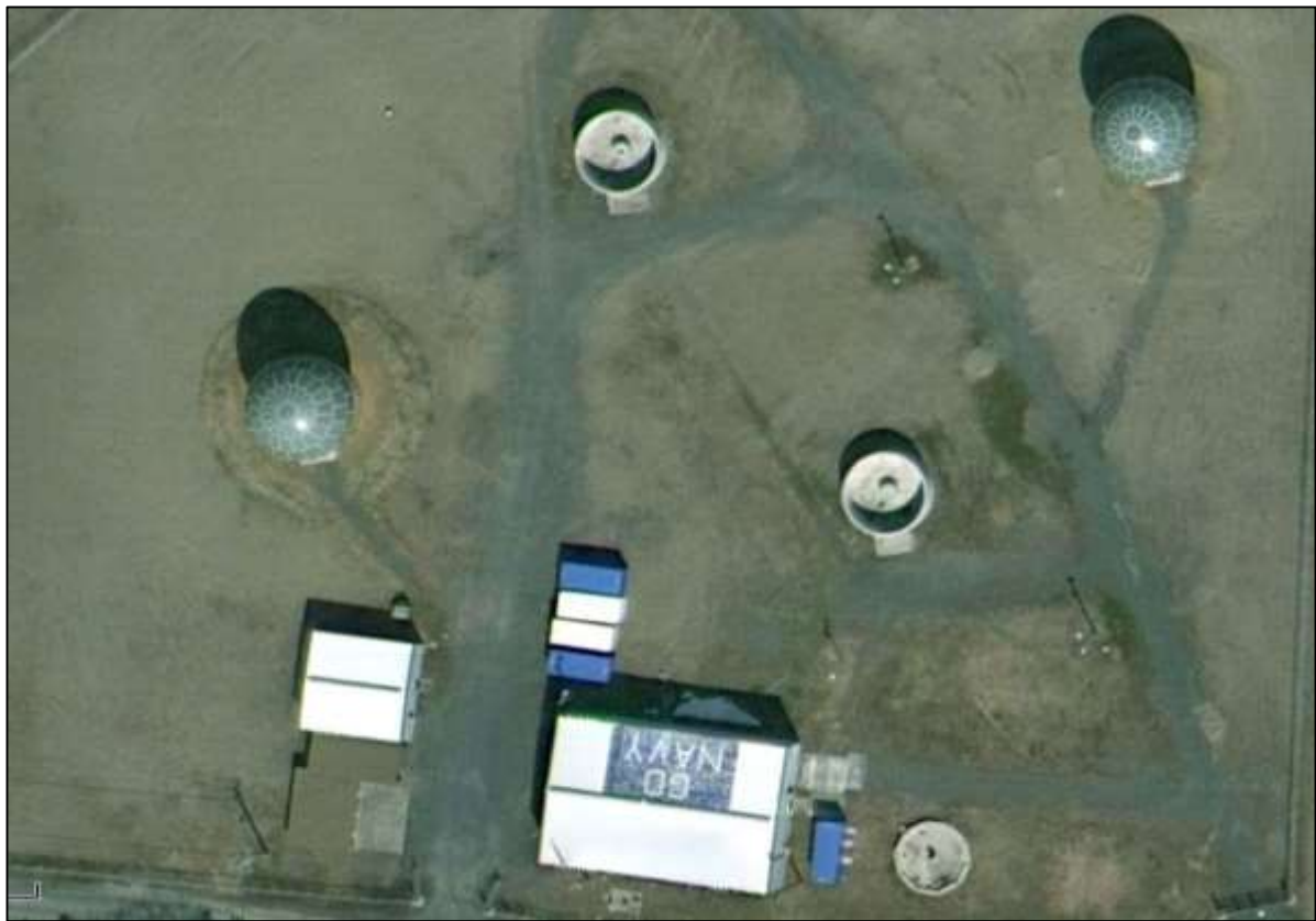
Plate 161 Project ICEbox (two radomes), Misawa, GoogleEarth imagery, 12 September 2012
