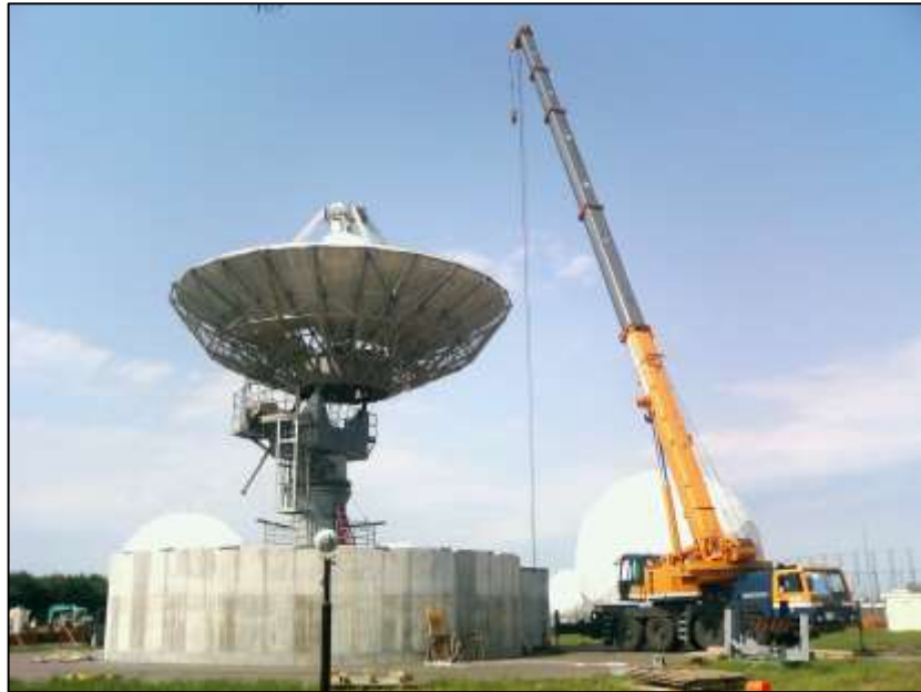
Plate 144 Installation of new dish/radome, Misawa, June 2007
