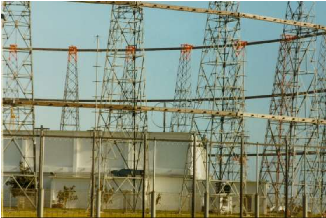
Plate 69 AN/FRD-10 CDAA at Camp Hanza, Okinawa, 27 April 1981 (Note loop DF antenna in centre)
