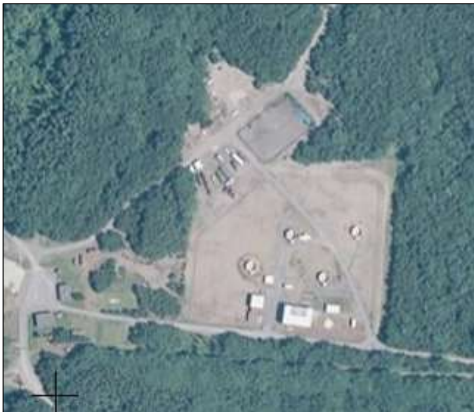
Plate 160 Project ICEbox (radomes dismantled), Misawa, 2008
