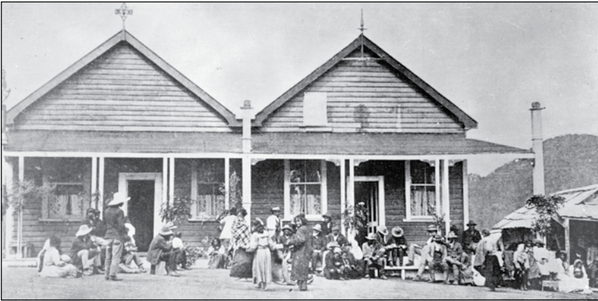
Rua Kenana's house, Hiruharama Hou (New Jerusalem), Maungapohatu, April 1908. One side was for Tuhoë, the other for Whakatohea, who were among the first to join him at Maungapohatu. Hiruharama Hou was modelled on the house that Solomon built with instructions from his father, thus invoking Christ's lineage as the Son of God, and Rua's lineage as king and messiah.
