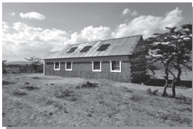
The school building with solar panels in the village of Empash
