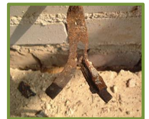
Old Wall Tie
