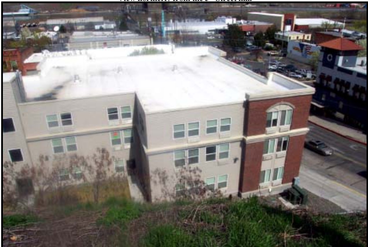
View north of the new building from the top of the steep hill to the south.
