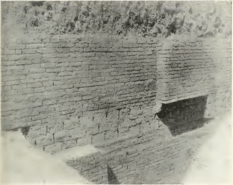
The Ziggurat on the northwestern side, near the northern corner. Below are visible the panelled walls of brick of Ashurbanipal. Above are seen the great blocks of unbaked brick of the last great Reconstruction. Above this are formless débris and very late walls.
