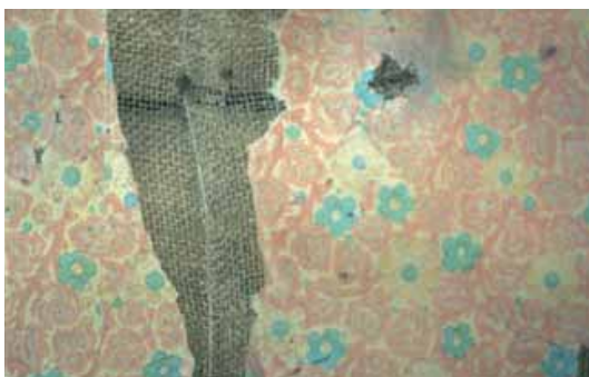
(75). Detalle del papel mural y su arpillera al interior de la Casa Stirling. Bahía Douglas, 1997- 2001 Detail of the wallpaper and its burlap in the interior of Casa Stirling. Douglas Bay
