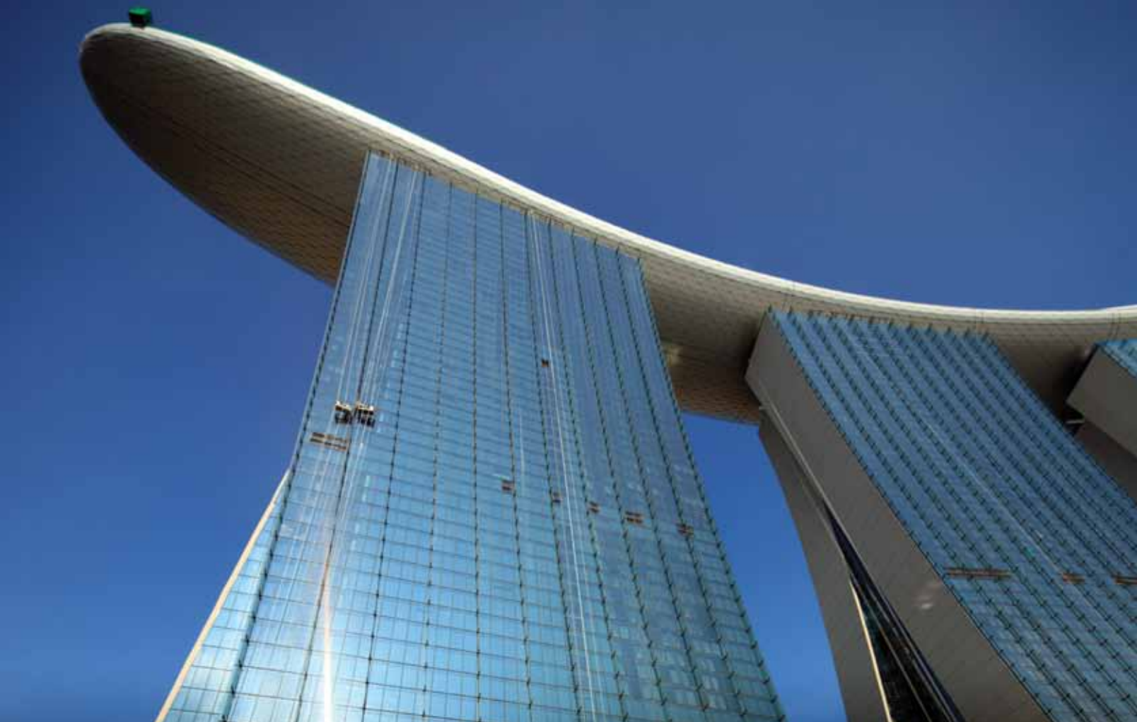
Figure 5: The SkyPark appears to float high above the hotel towers. With a cantilever of 218 feet, the roof deck is the longest habitable cantilevered observation deck in the world. Courtesy of Arup.
