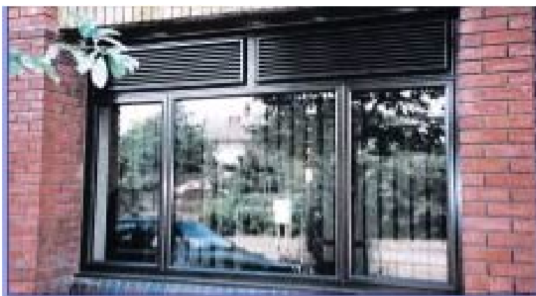
Figure 2: Facade Ventilation devices
