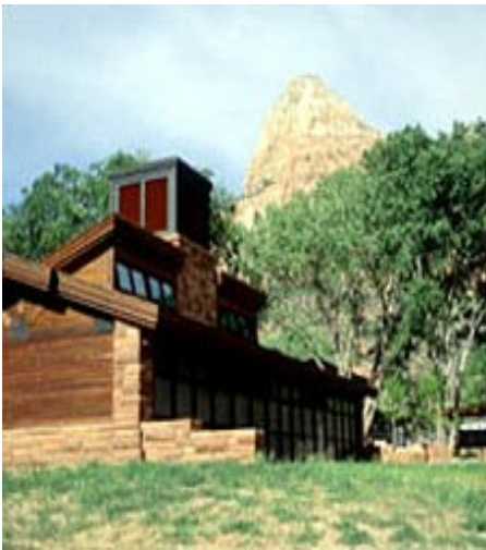
Figure 3: Photo of the Visitor Centre showing cooling tower and high windows for exhaust air
