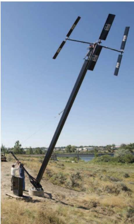
Photo on left: Blackhawk tilt-rotor vertical-axis wind turbine installed at Idaho National Laboratory's Center for Advanced Energy Studies.
