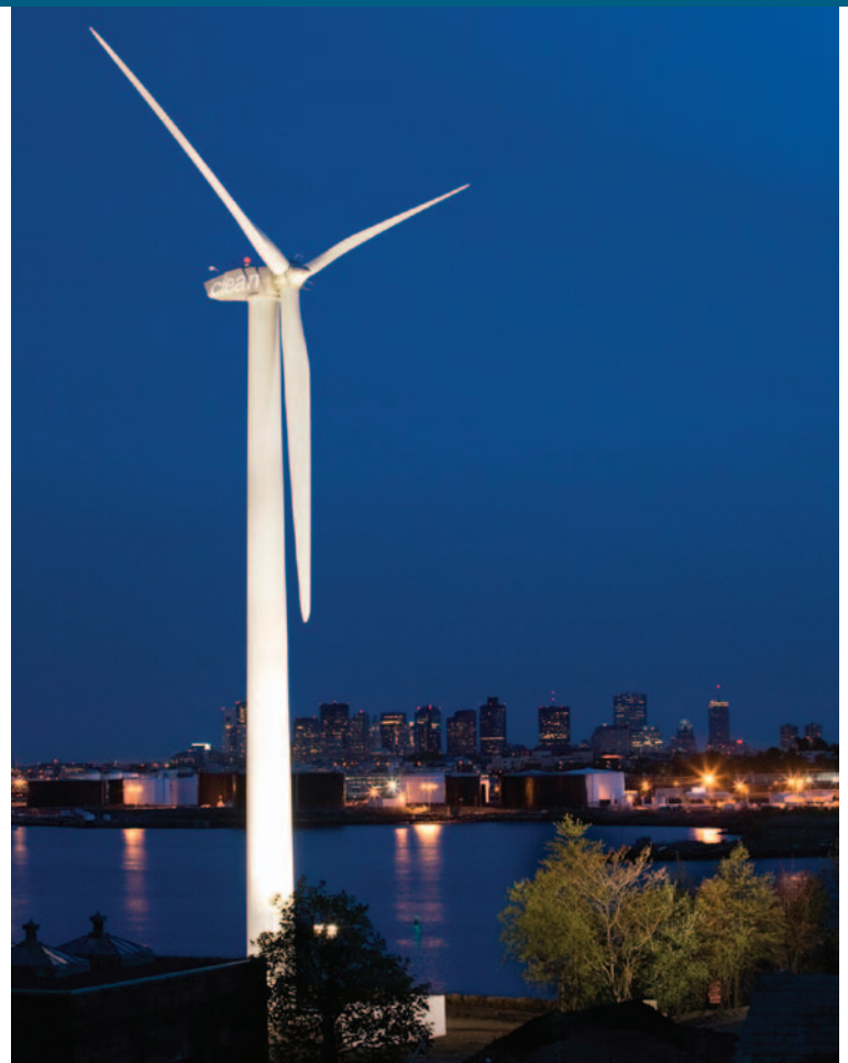
A 600-kilowatt wind turbine installed near Boston, Massachusetts.
