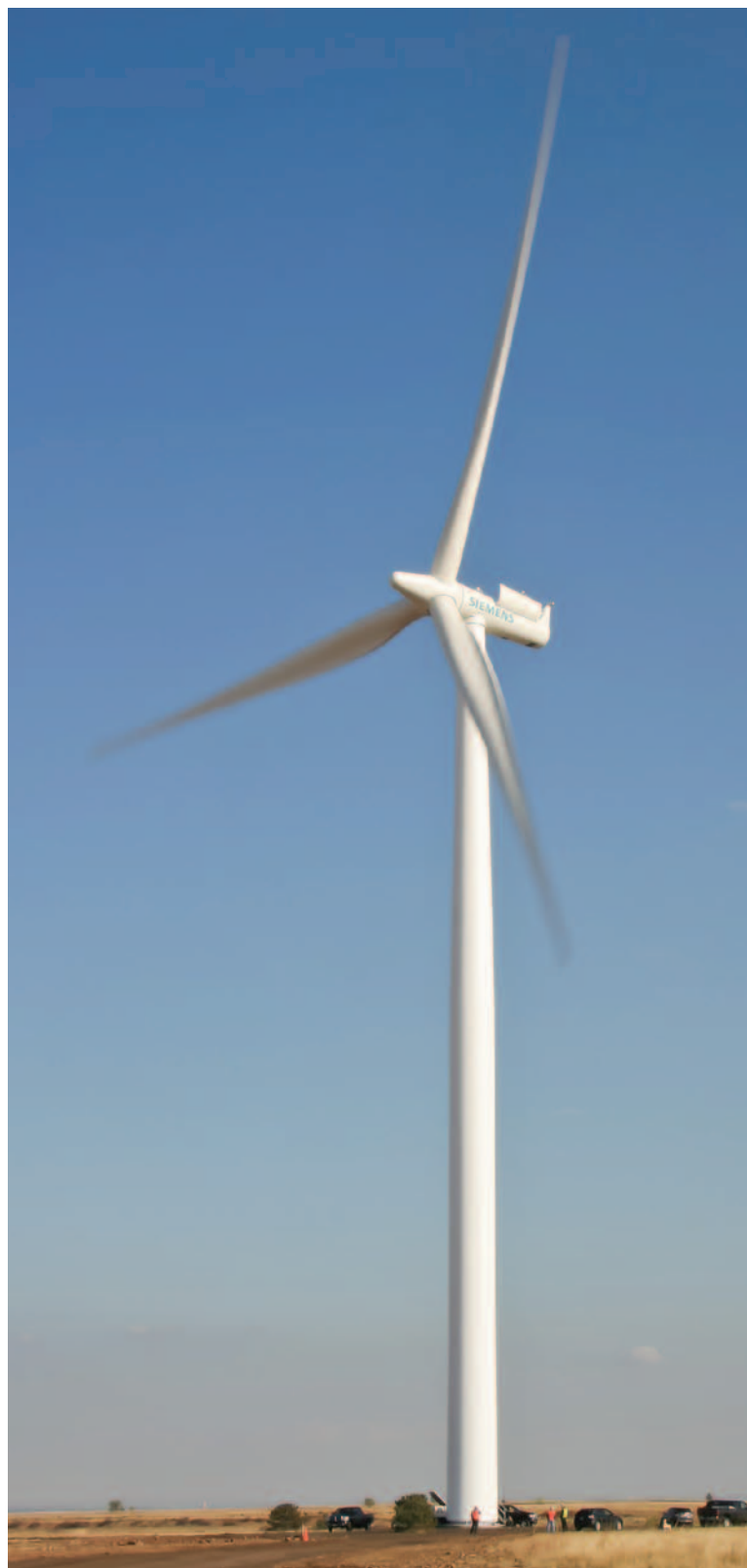
The 2.3-megawatt Siemens wind turbine installed at the National Renewable Energy Laboratory is the centerpiece of a government-industry research partnership between Siemens and the laboratory to study the turbine's performance and aerodynamics.
