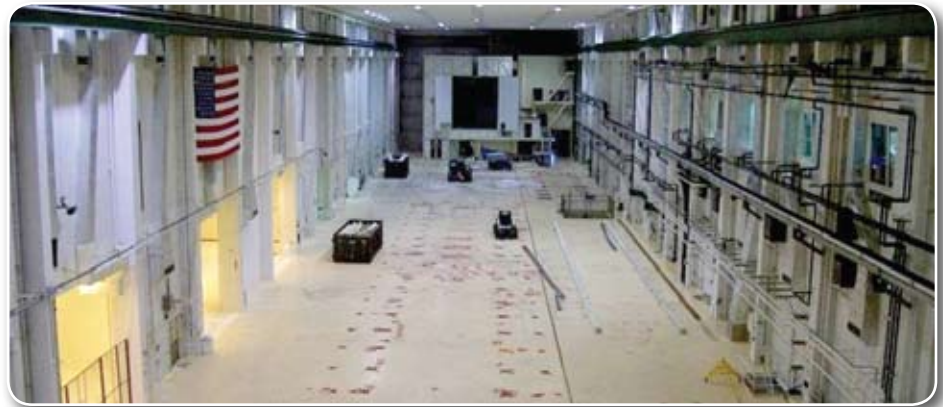
Above: Kennedy Space Center's Operations and Checkout Building high and low bays were prepared for complete ceiling-to-floor renovation.
