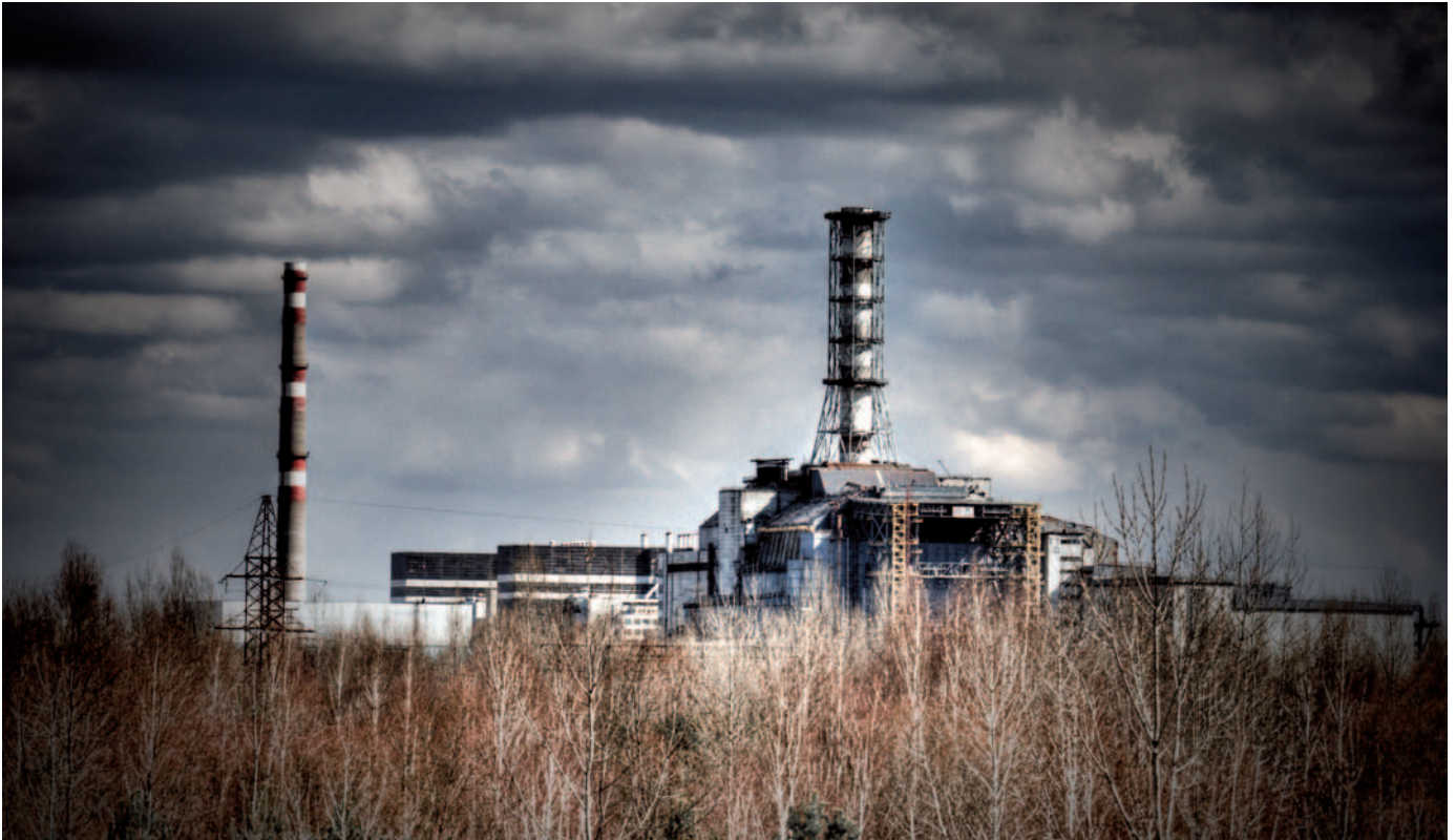
Ghost from the past: encased in crumbling concrete, the deadly contents of Chernobyl's reactor number 4 still exert a far-reaching effect on the area.
