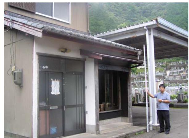
Photo.8 Jizo-an Temple, Kii-nagashima town. The tsunami wave at the 1854 Ansei tsunami went up to 60cm lower than the rafter of the building.
