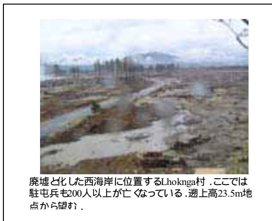
Photo. 2 Damaged area due to 23.5m tsunami inundation in Aceh.
