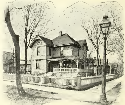
RESIDENCE OF T. F. AXELL
