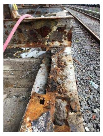
Platform Steel deterioration
