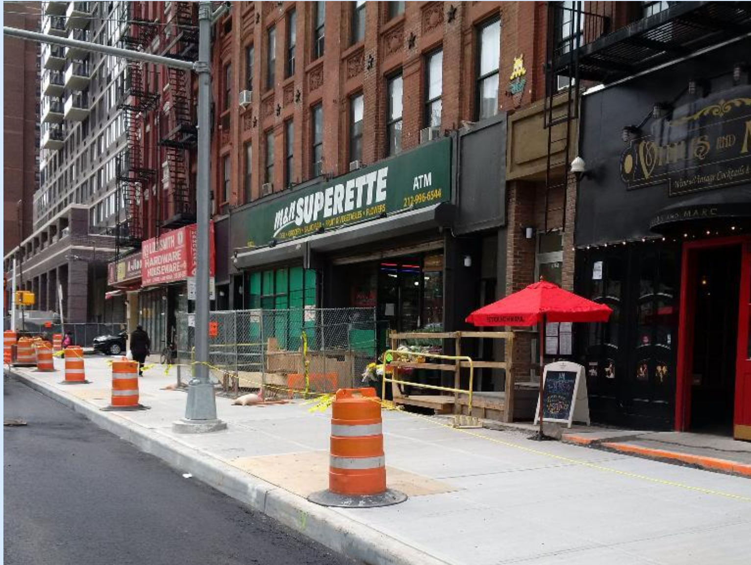
Sidewalk restoration west side of 2 nd Avenue between 94 th - 95 th Streets
