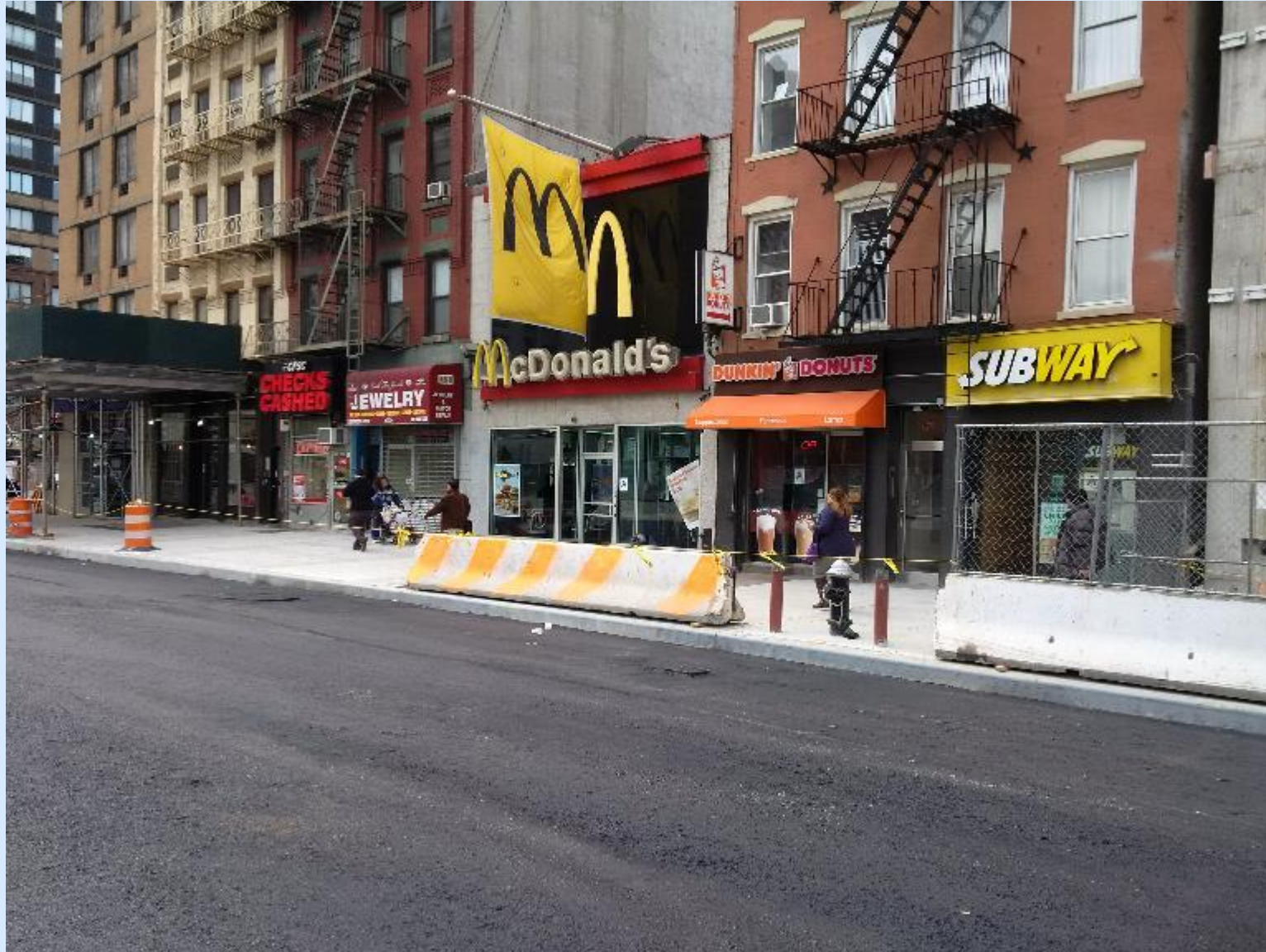
Sidewalk restoration west side of 2 nd Avenue between 96 th - 97 th Streets
