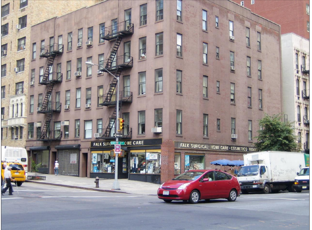
View of northwest corner of 72nd Street and Second Avenue 5
