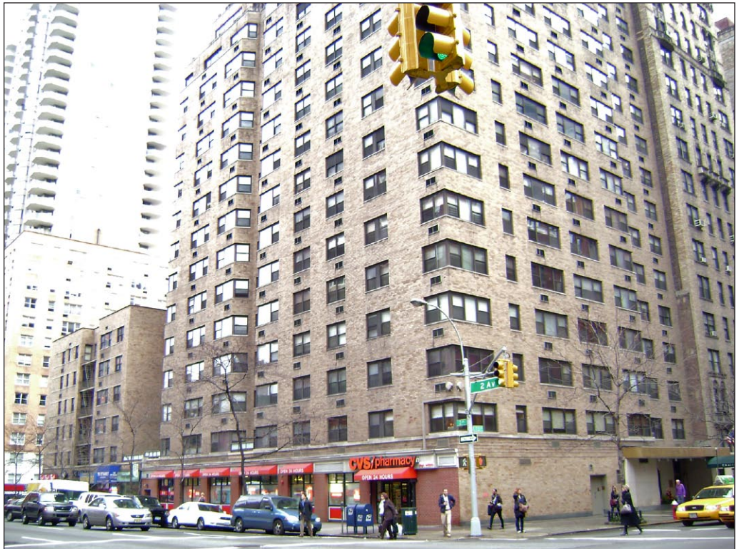
View of northeast corner of 72nd Street and Second Avenue 2
