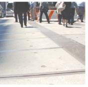
vertical walls and a frame is built to support concrete or metal street decking (1). The decking allows the street to remain open to traffic and pedestrians while excavation and construction continue in the tunnel below.
