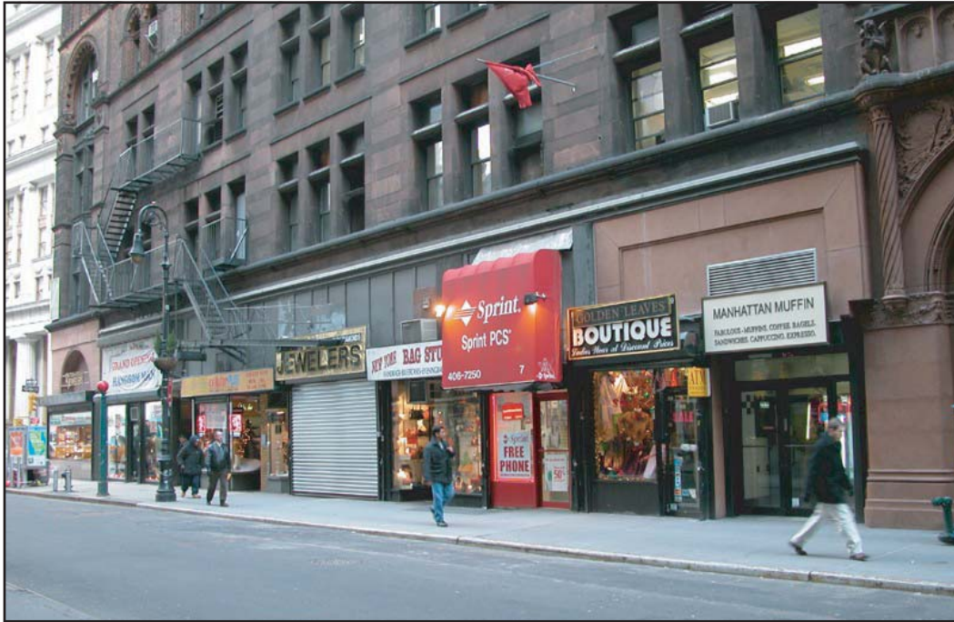
Figure 3-5: Corbin Building seen from John Street under Alternative 9
