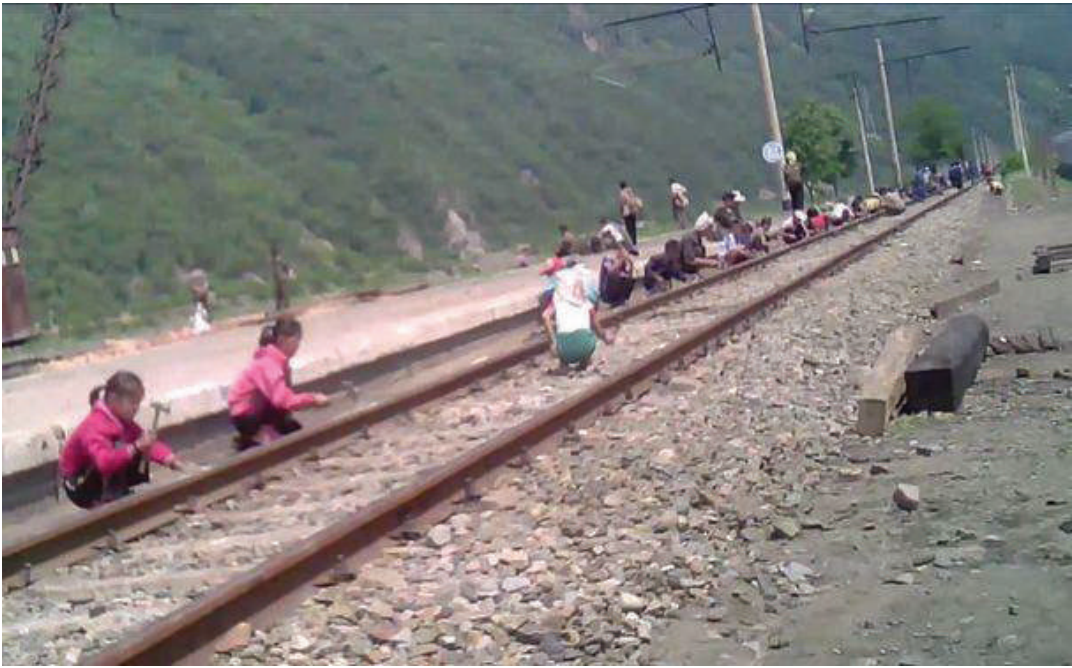
Figure 8 41 - Spreading gravel over the railroads.
