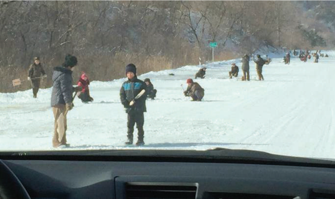
Figure 15 58 - Young children, using inadequate tools to clear the snow-covered roads.
