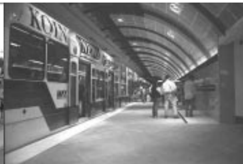
Tunnel (Portland, OR)
